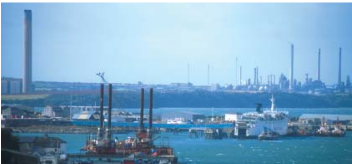
Milford Haven port – over 90% of UK overseas trade is carried by sea Photographer Paul Kay
